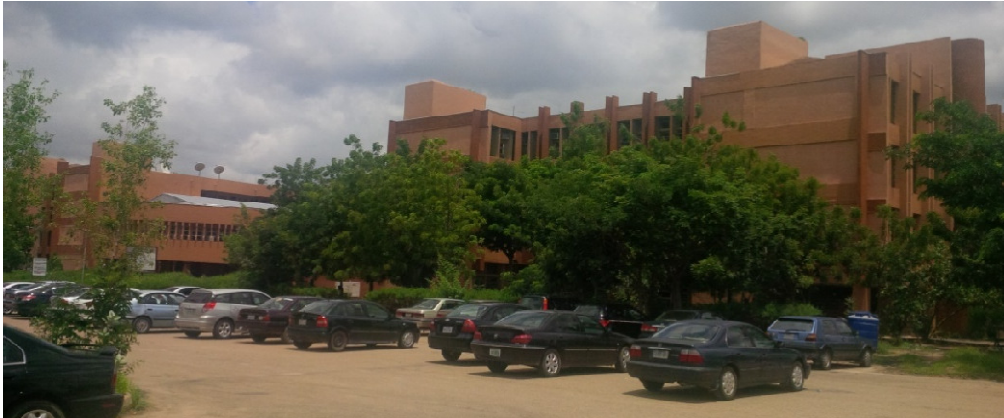
Plate 1. Federal secretariat building, Bauchi, Bauchi State, Nigeria (Field survey, 2014)
