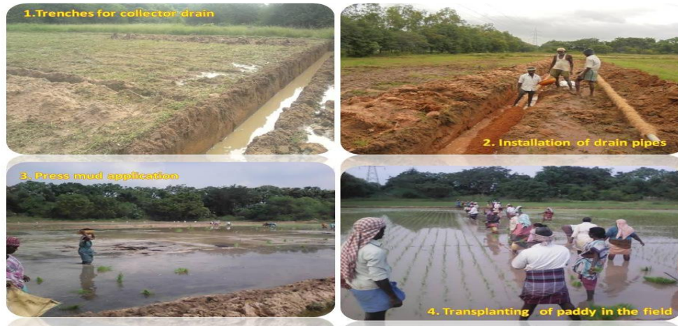
Plate 1. Installation of controlled drainage
