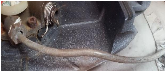
Fig. 9. High pressure pipe
