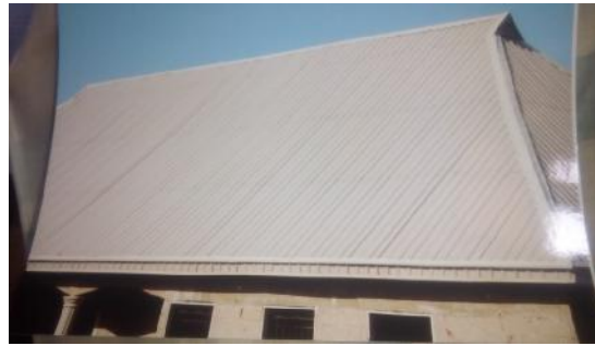
Fig. 3. Corrugated (coloured) roofing sheet (zinc)
